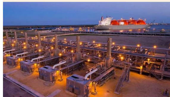
Cheniere Energy's LNG plant at Sabine Pass
